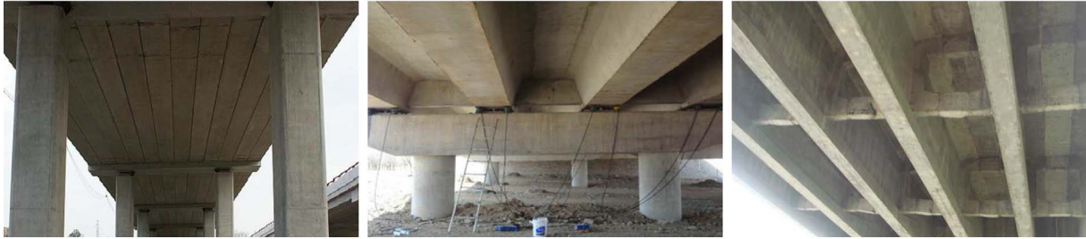
(b) The real images of three different types of typical bridges
